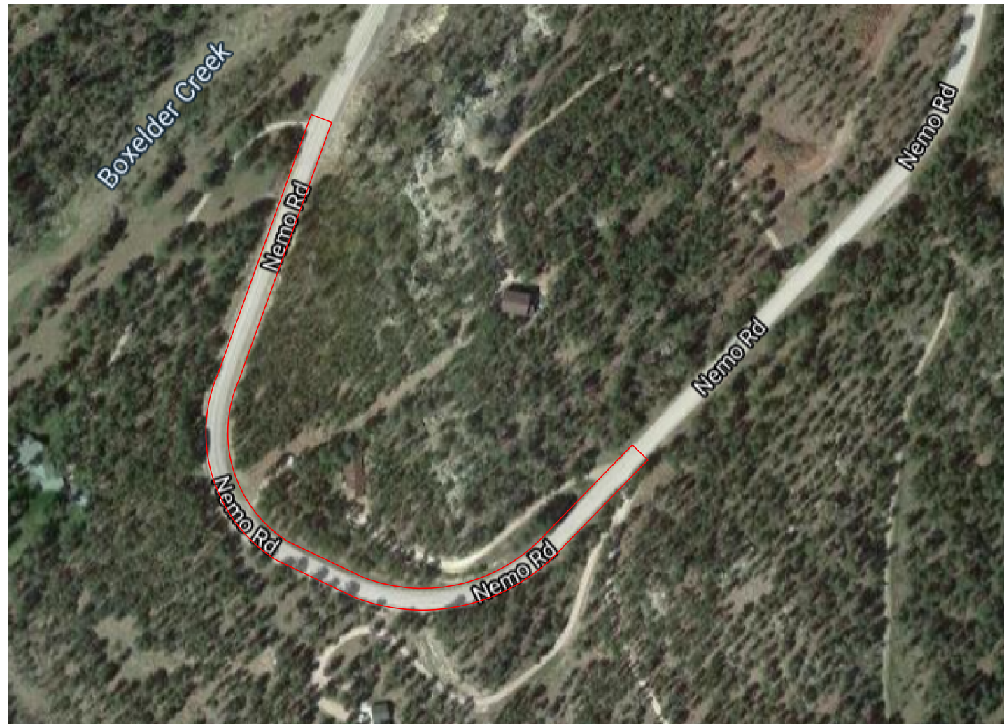
Nemo Road (0.28 mile) - Switchback curve approximately 0.75 mile east of Norris Peak
