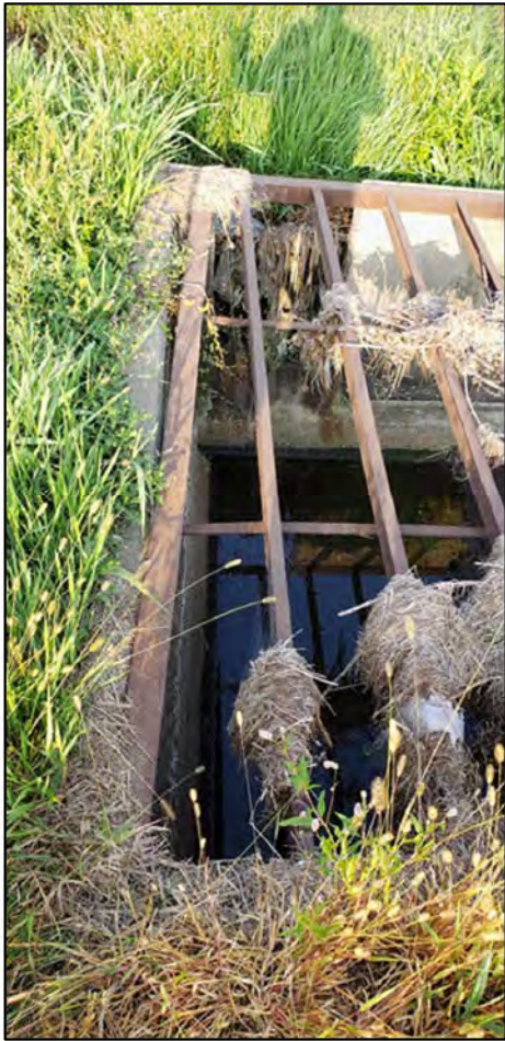
STA. 59+28 LOW FLOW CUTOUT OF 9' X 20' INLET
