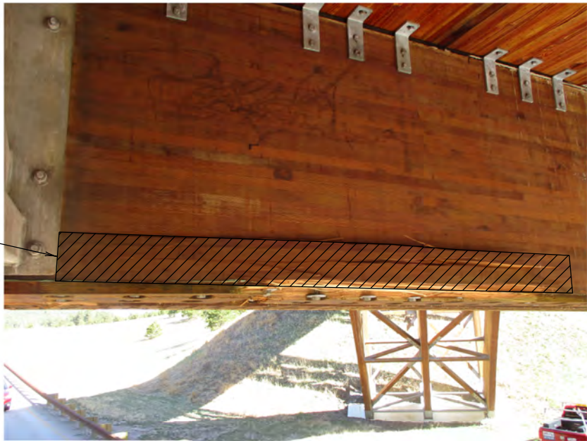
GIRDER 3 GLULAM REMOVAL (Showing Gluelam Removal Only)
