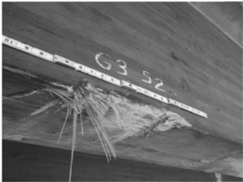
TYPICAL GIRDER DAMAGE
