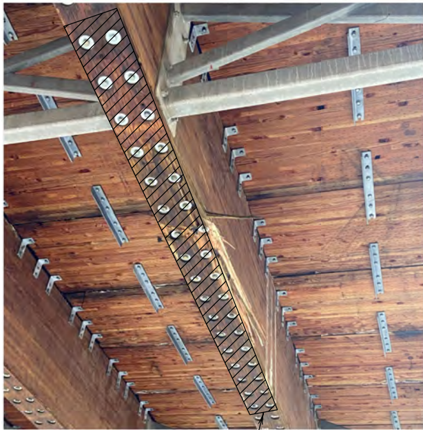
GIRDER 3 BACKER BOARD REMOVAL (Showing Backer Board Removal Only)
