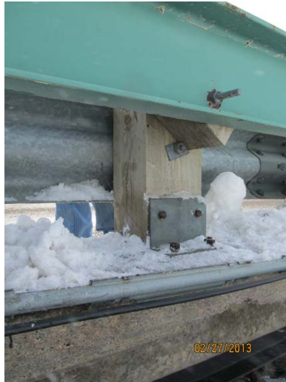
Fig 3 – Typical bolting arrangement – looking at the backside of wood blocks and steel channel
