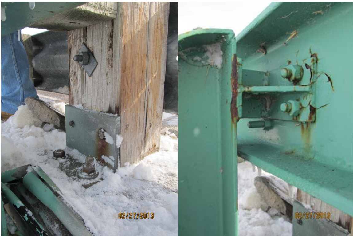
Fig 1 & 2 – Typical bolting arrangement at steel channel posts ("blind posts") – looking at the backside of steel channel and wood blocks
