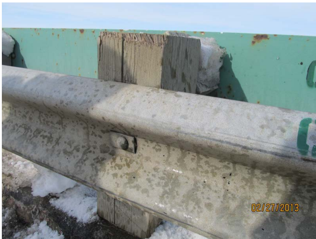
Fig 4 – Typical view of the front side of the blocks and W beam guardrail
