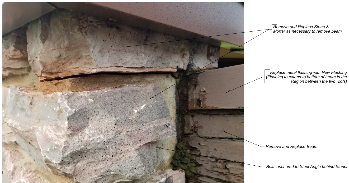
WEST PICNIC SHELTER (Looking West at beam embedded in Stone Wall)
