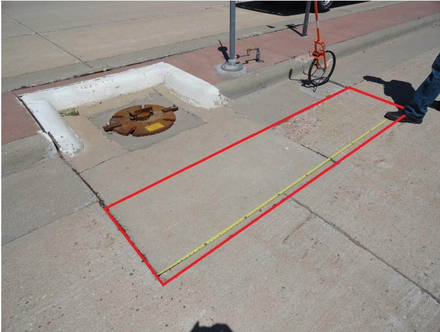
Detail of additional removal – approximately 2.5' x 9.5' (~23.8 sq ft)
