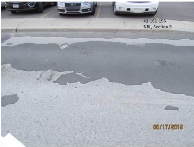
TYPICAL SPALL
