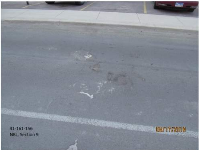
TYPICAL SPALL
