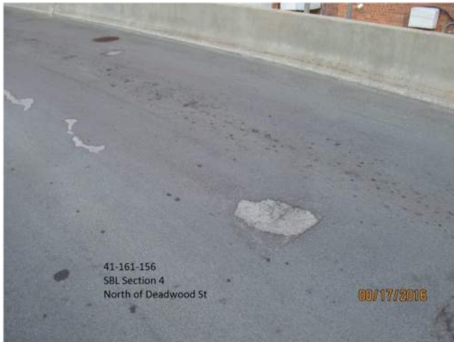
TYPICAL SPALL
