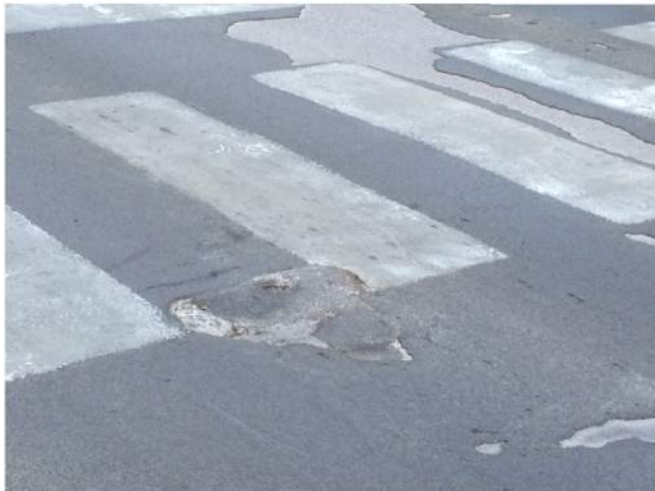
TYPICAL SPALL
