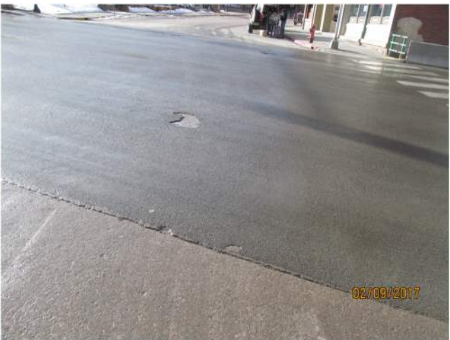
TYPICAL SPALL
