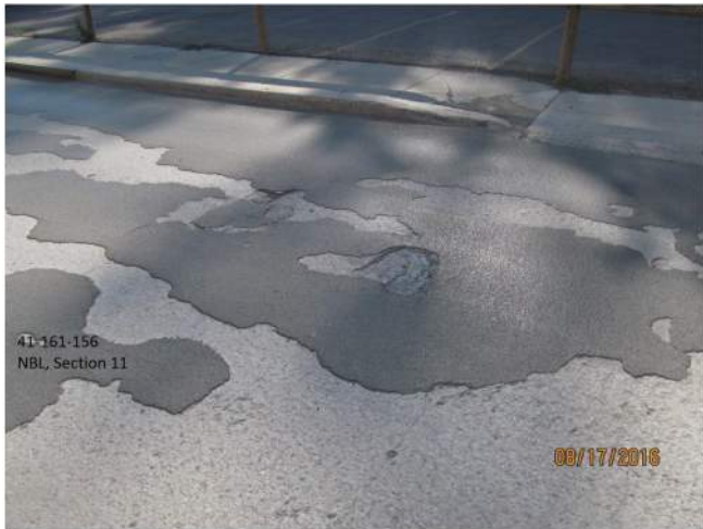
TYPICAL SPALL
